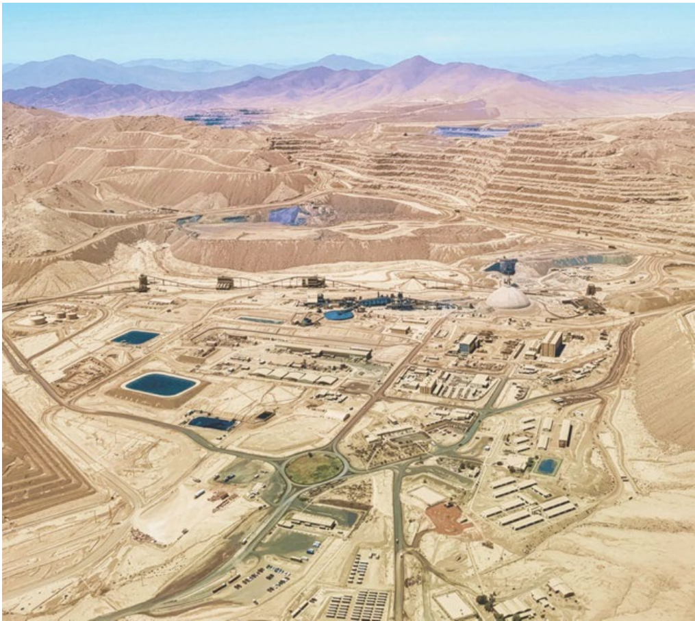
The Mantoverde pyrite plant site.
