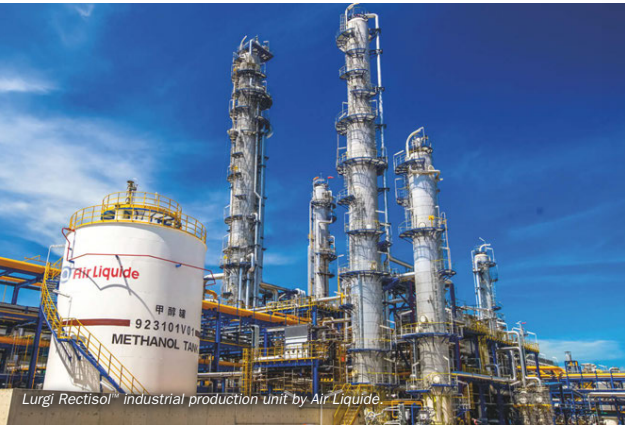
PHOTO: AIR LIQUIDE
