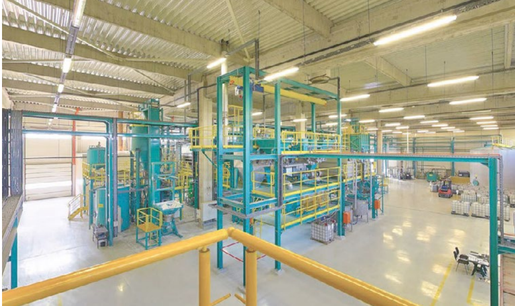
Innovation: Prayon Technologies proved its magnesium removal process at the company's Technophos semi-industrial demonstration plant, Varna, Bulgaria.
