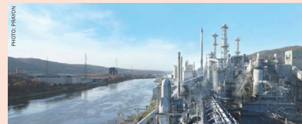
Prayon's state-of-the-art Engis phosphate production complex in Belgium.
