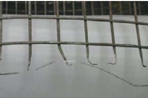
Photo 7: Corroded cage wires at the bottom.
