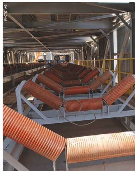
The interior of Mosaic's new large-scale precision blending plant at Tocantins, Brazil, showing conveyor installation during the construction phase.
