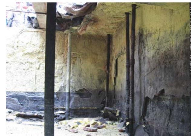
Fig. 1: Sulphur pit roof and wall failure due to lack of maintenance bringing down sulphur containment in a sulphur recovery unit at a Southwest USA petroleum refinery
