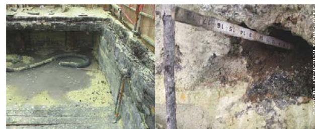
Fig. 5: Sulphur pit sidewall leaking steam coil penetrations resulting in concrete degradation and reduced molten sulphur heating efficiency.
