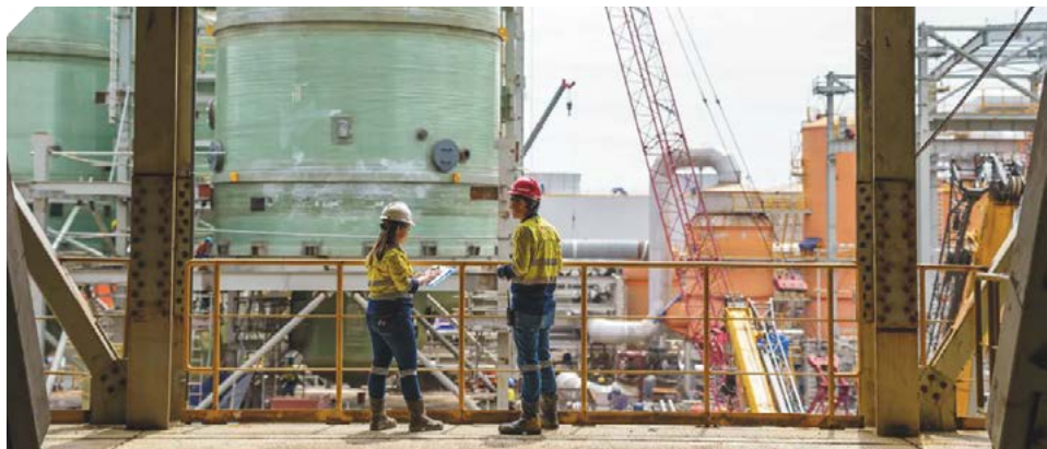
Construction work at the Merkada pyrite plant, Indonesia.
