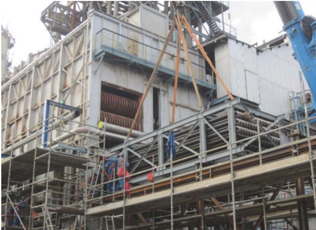
Fig. 6: Saturator coil installation.
