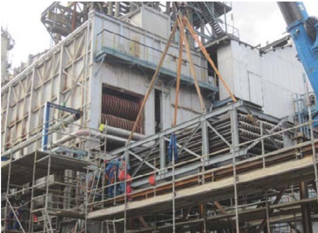
Fig. 6: Saturator coil installation.
