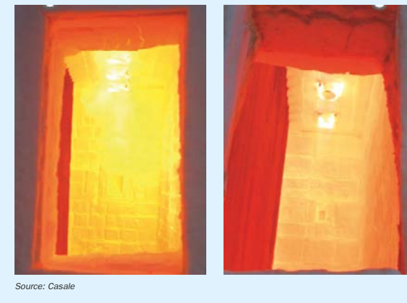
Fig. 3: Burner behaviour before (left, with flame distortion) and after revamping (right, showing normal flame appearance)
