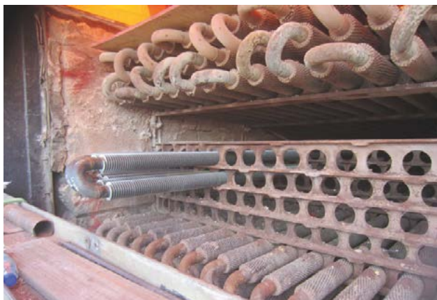
Fig. 7: Recoiling the convection section reusing existing tube sheets.
