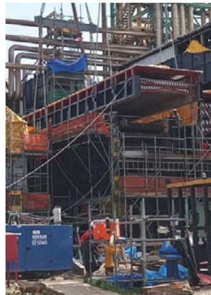
Fig. 5: Complete convection section revamping, including steam superheating coils (hot and cold) supplied as completed modules.
