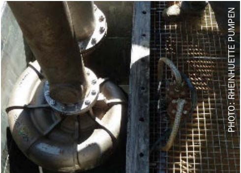
The vertical pump is installed in the tank of the sulphuric acid plant.
