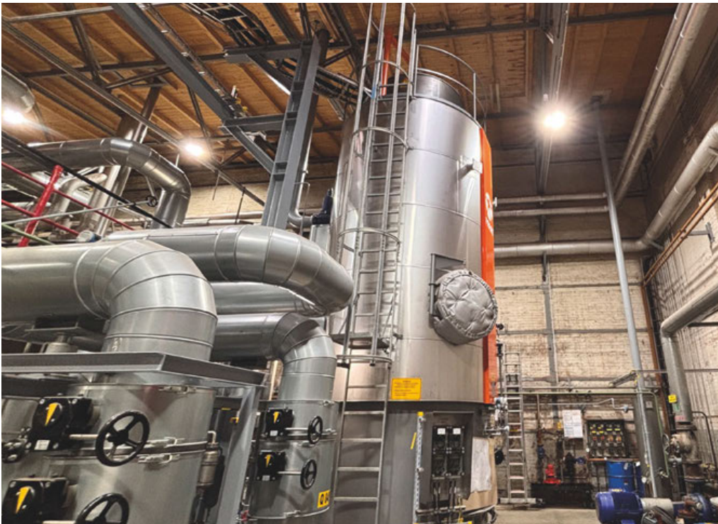
Renewable power-to-heat boiler at K+S’s Neuhof site. It can produce up to 26 tonnes of process steam per hour when operating at full power.
