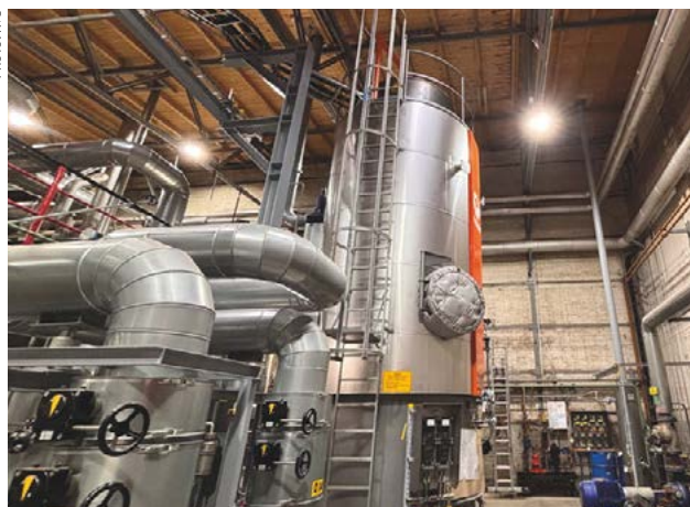
Renewable power-to-heat boiler at K+S's Neuhofer site. It can produce up to 26 tonnes of process steam per hour when operating at full power.
