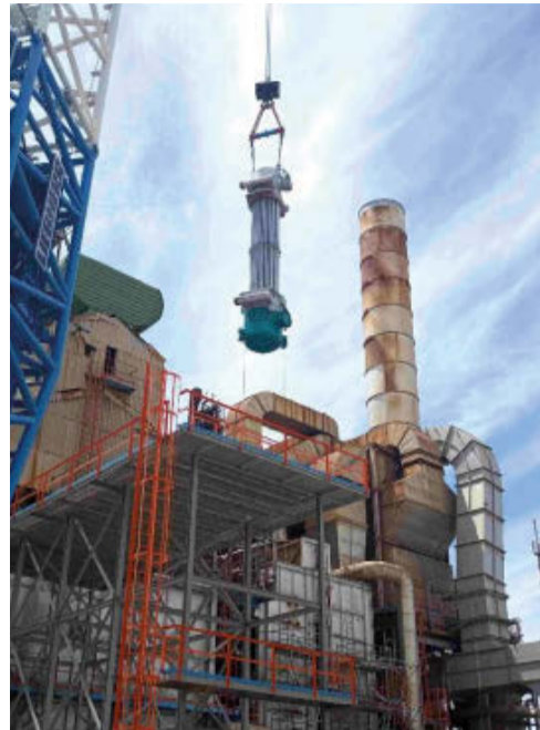
Fig. 4: Lifting 1101-C into place.
