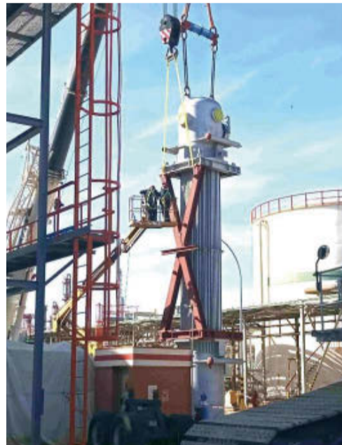
Fig. 7: Reinforcing frame dismantling.
