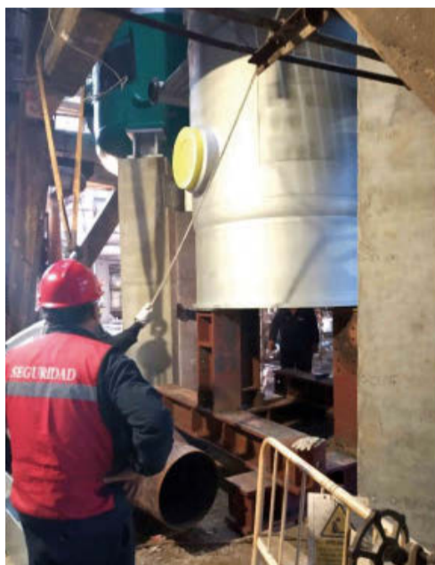
Fig. 9: 1102-C on temporary support.
