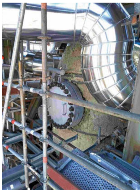
Fig. 12: Insulation in progress.
