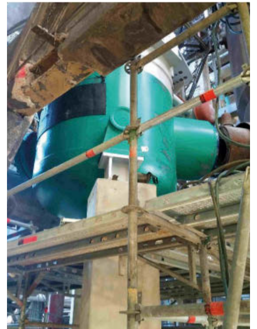
Fig. 5: Placing 1101-C onto foundation.
