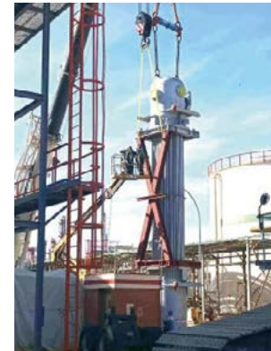
Fig. 7: Reinforcing frame dismantling.
