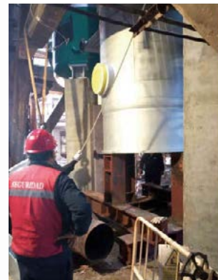
Fig. 9: 1102-C on temporary support.
