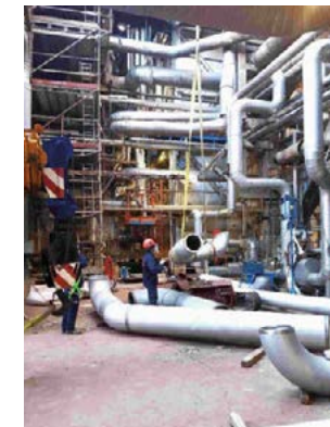
Fig. 11: Prefabricated spools.
