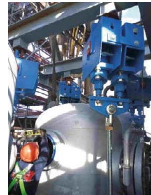
Fig. 10: 1102-C hanging on spring supports.
