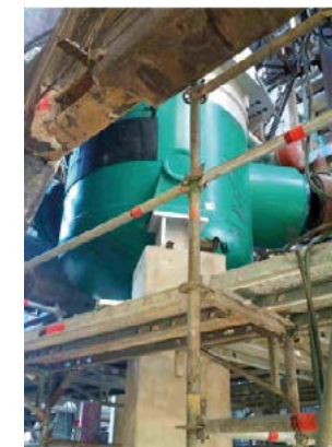
Fig. 5: Placing 1101-C onto foundation.
