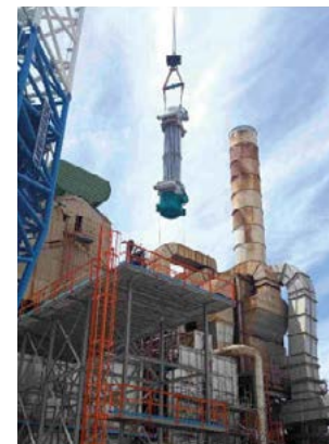
Fig. 4: Lifting 1101-C into place.
