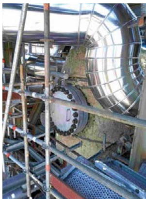
Fig. 12: Insulation in progress.
