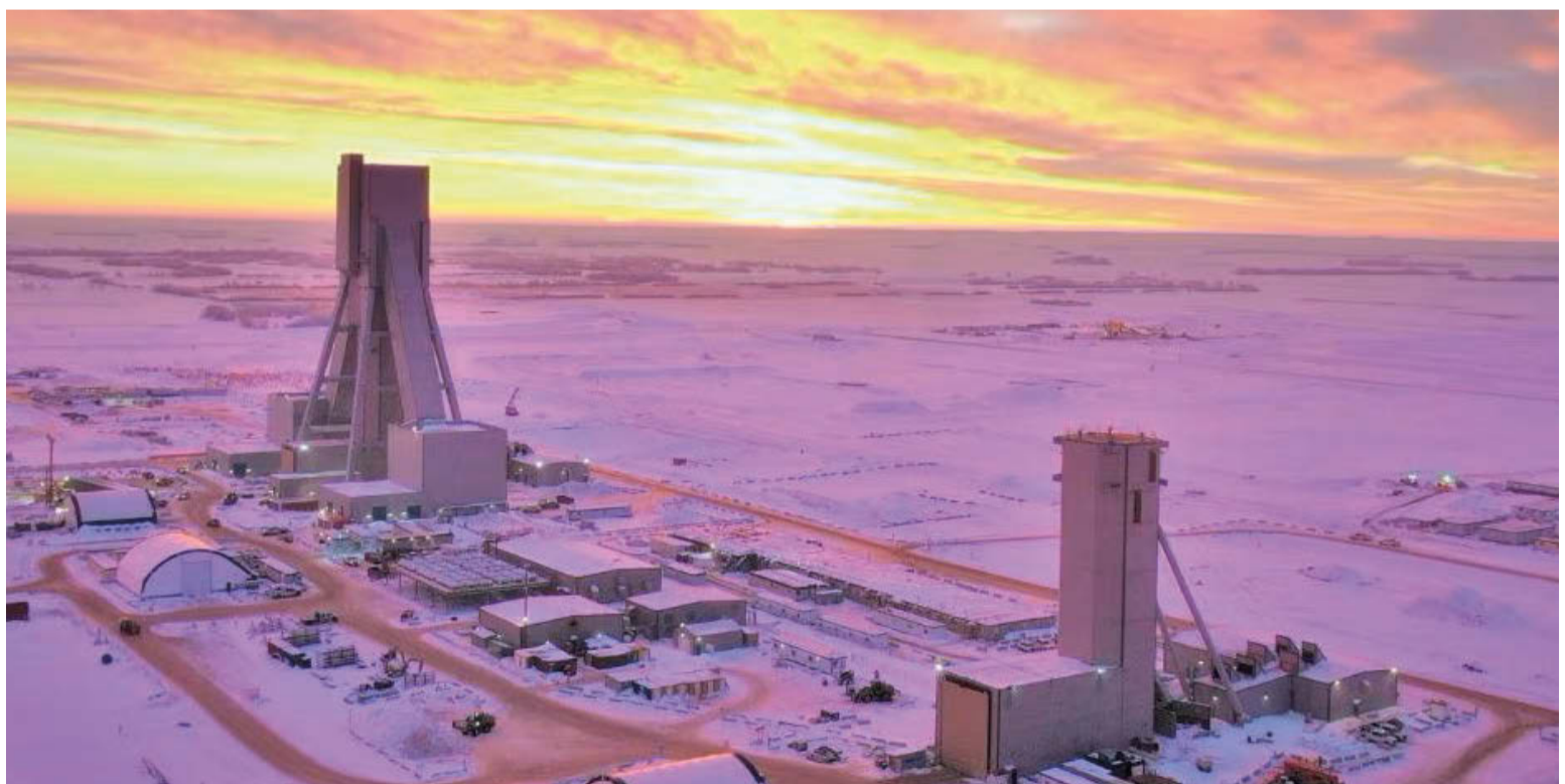
The 4.35 million t/a capacity Jansen S1 project is expected to produce its first potash ore towards the end of 2026, following a six-year construction phase. The project is located 140 kilometres east of Saskatoon, Saskatchewan.
