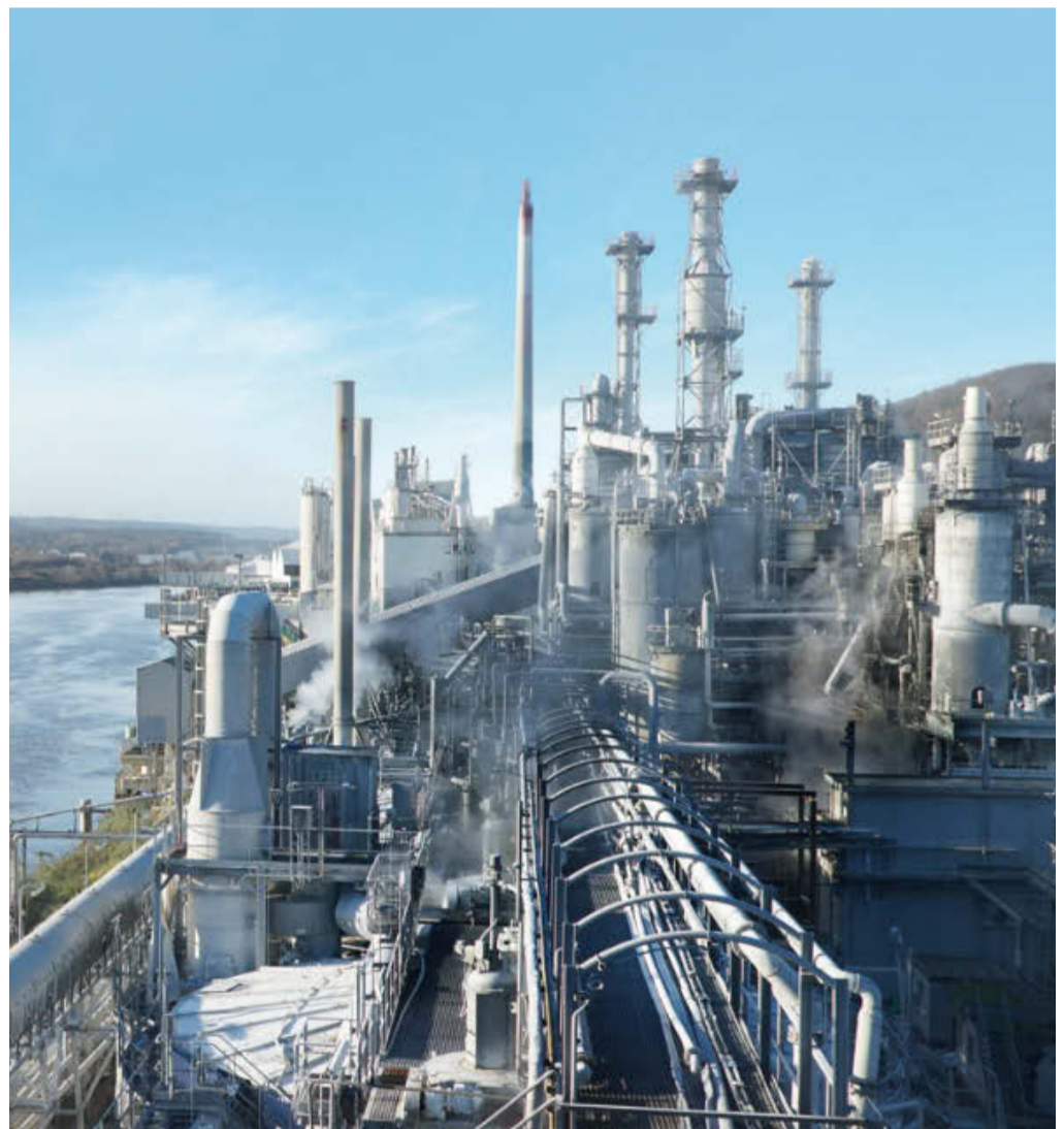
Prayon's phosphate production complex at Engis in Belgium.
