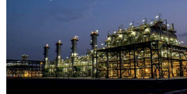
The Shah processing plant, Abu Dhabi.
