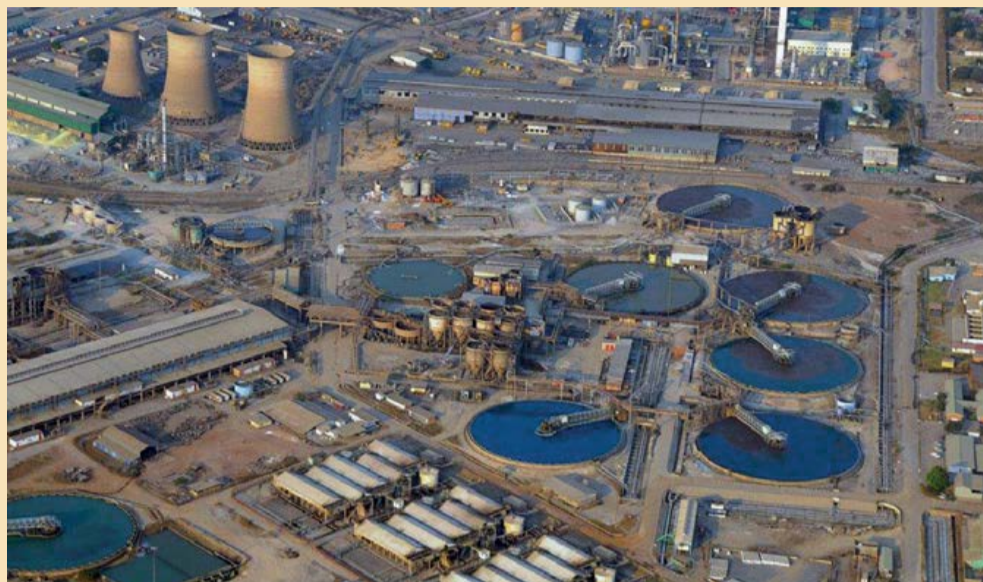
Tailings leach plant at KCM.
