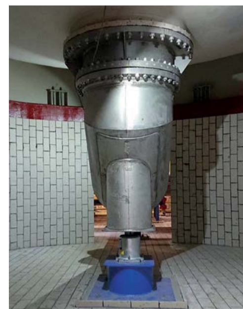
Acid piping fabricated in NORAM SX™ alloy.
