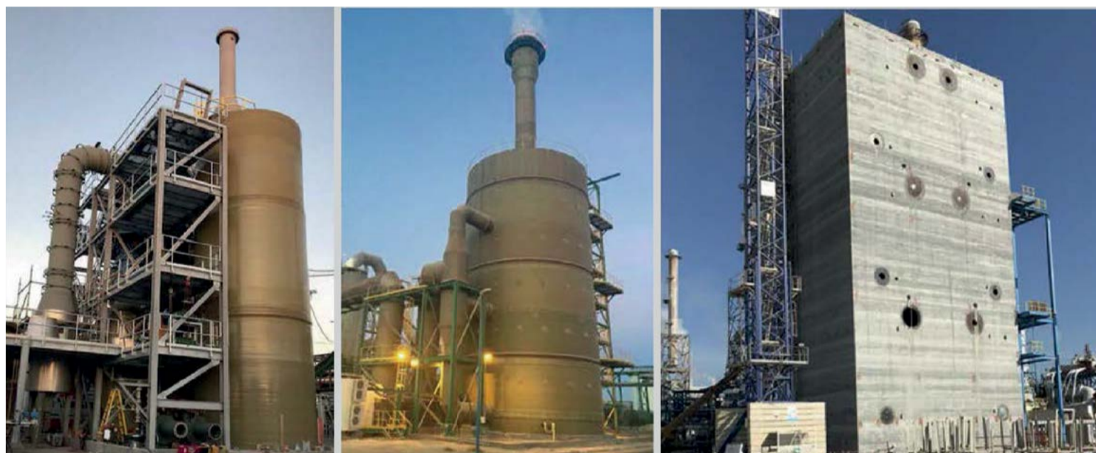
Examples of Sulfacid® industrial installations.
