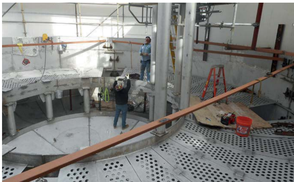
Assembly of a NORAM converter in SS304H.
