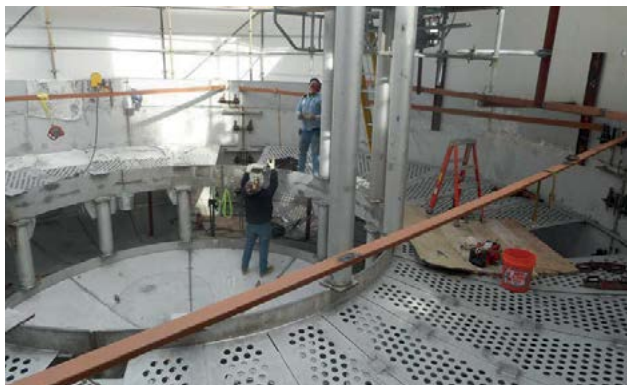
Assembly of a NORAM converter in SS304H.
