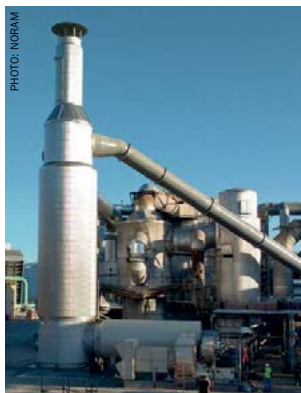
NORAM preheat gas exchanger fabricated in SS304H.
