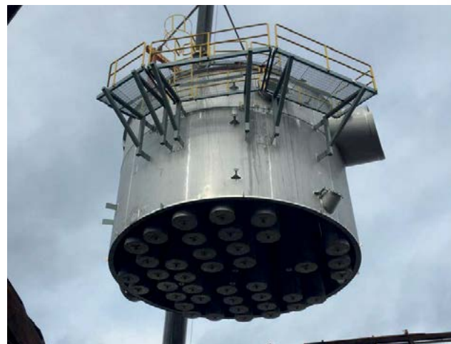
Installation of a MECS® ZeCor® alloy acid tower
