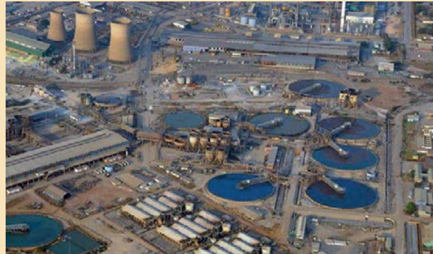
Tailings leach plant at KCM.
