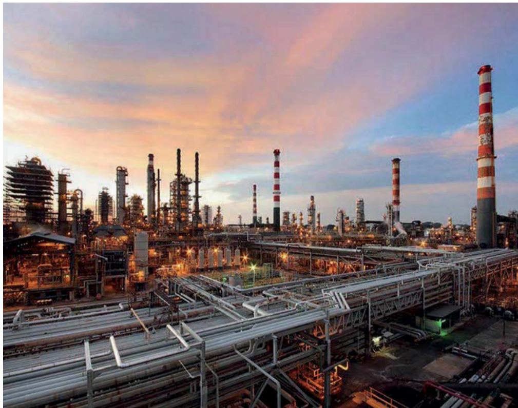
ExxonMobil's Jurong refinery at Singapore.
