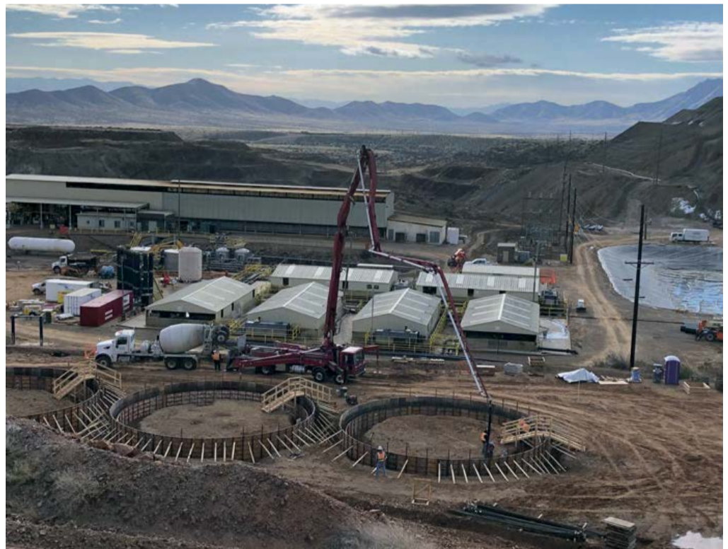
Acid storage area construction at the Gunnison Copper Project.
