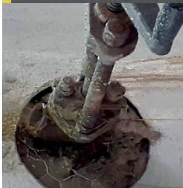
Fig. 5: Strahman sampling valve
