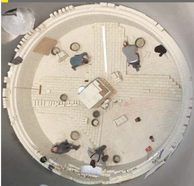
Fig. 6: Tower brick lining work
