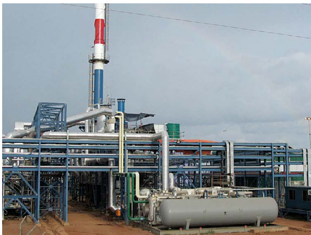
Sulphuric acid plant with integrated liquid \text{SO}_2 production.
