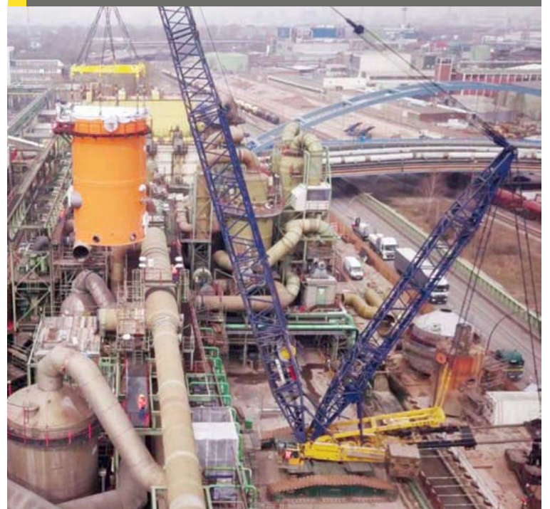
Fig. 7: Lifting the new tower in to place
