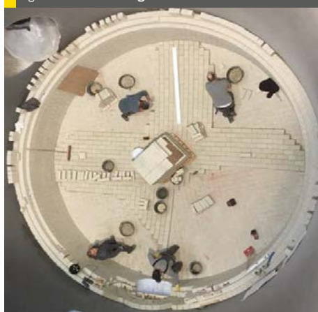
Fig. 6: Tower brick lining work
