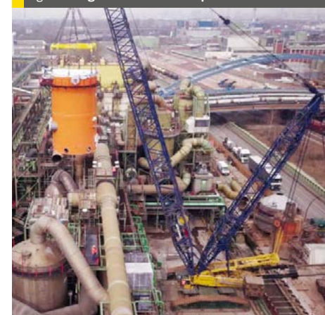
Fig. 7: Lifting the new tower in to place
