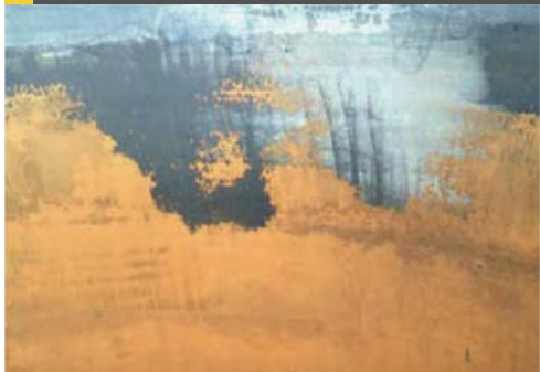
Fig. 10: Typical interior shell/roof surface with light coating of rust
