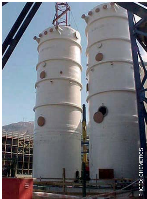
Fig. 2: Chemetics quench and scrubber venturi with variable throat design.
