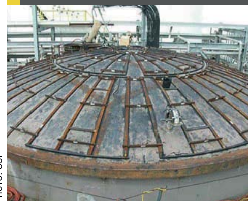
Fig. 4: ControTrace tank roof heating
