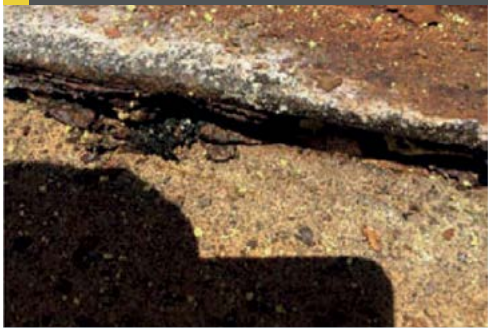
Fig. 9: Corrosion and scale under tank chime
