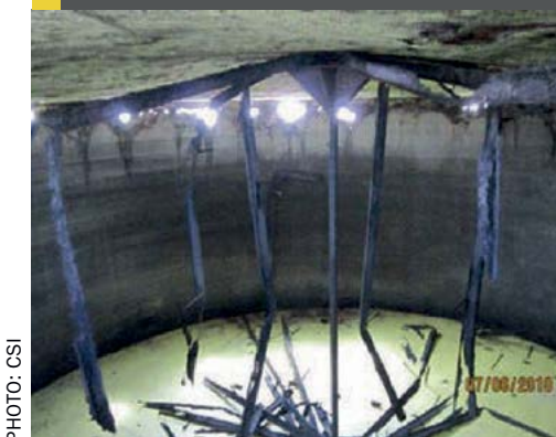
Fig. 3: Sulphur tank structure corrosion
