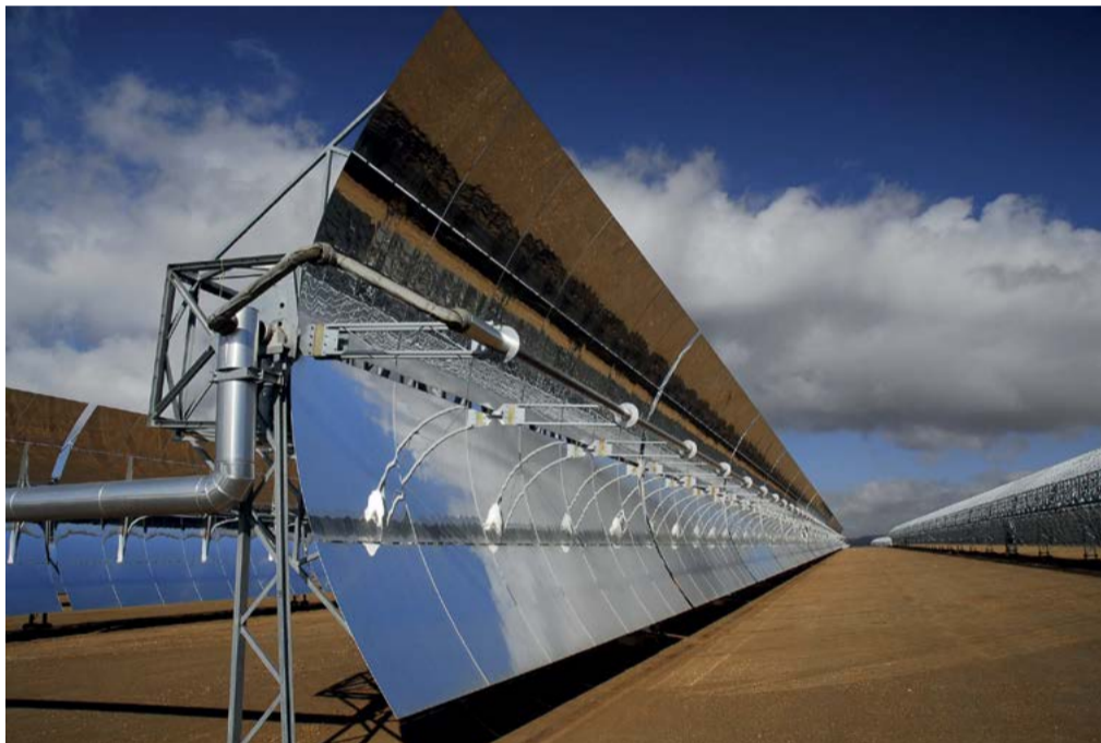
Fig. 1: Trough-shaped parabolic reflector.
