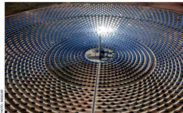
Fig. 3: Power tower with heliostats.
