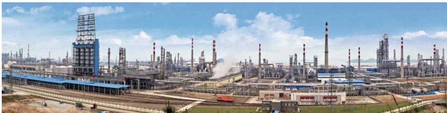
Fig. 5: CNOOC Huizhou Refinery in Guangdong, China.
