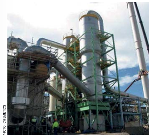
Fig. 2: New Chemetics SARAMET ® acid towers with modelling process design confirmed using plant operational data.
