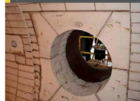
Fig. 13: Pre-formed bricks around manhole
