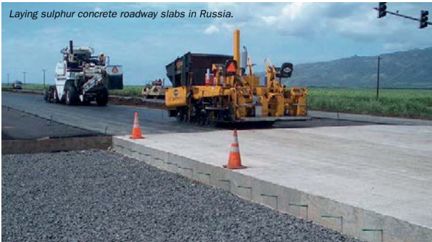
Laying sulphur concrete roadway slabs in Russia.
