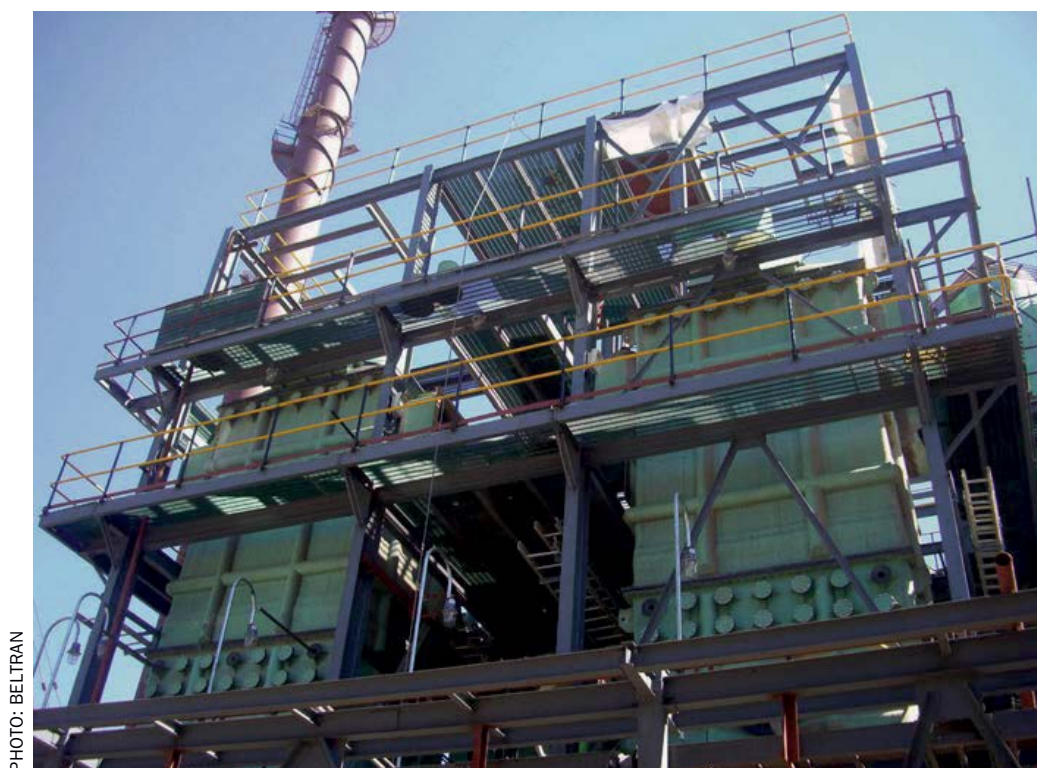
Fig. 6: Hindustan Zinc Ltd installed wet ESPs engineered by Beltran Technologies Inc. to control smelter emissions and effectively capture and remove fine sub-micron size particulate matter.
