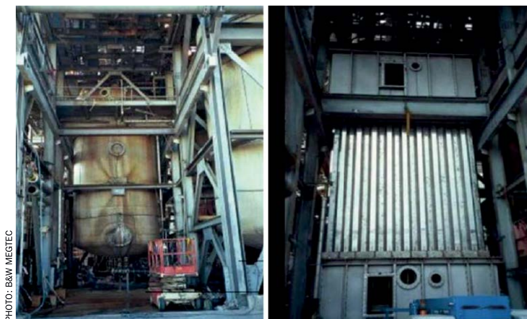
Fig. 5: Old lead wet ESP (left) to be removed and new alloy set ESP replacement (right) installed into existing structure (compact design provides more wet ESP performance per footprint).
