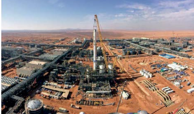
The Umm Wu'al phosphate plant under construction.
