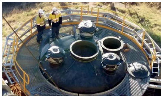
Fig. 10: Top of wet ESP with platform.
