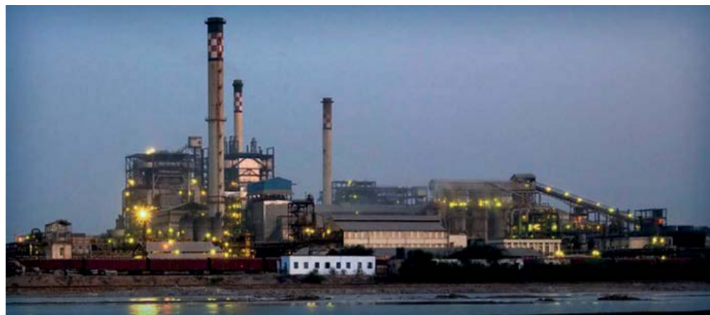
Tata Chemicals' fertilizer plant in Haldia, West Bengal.
