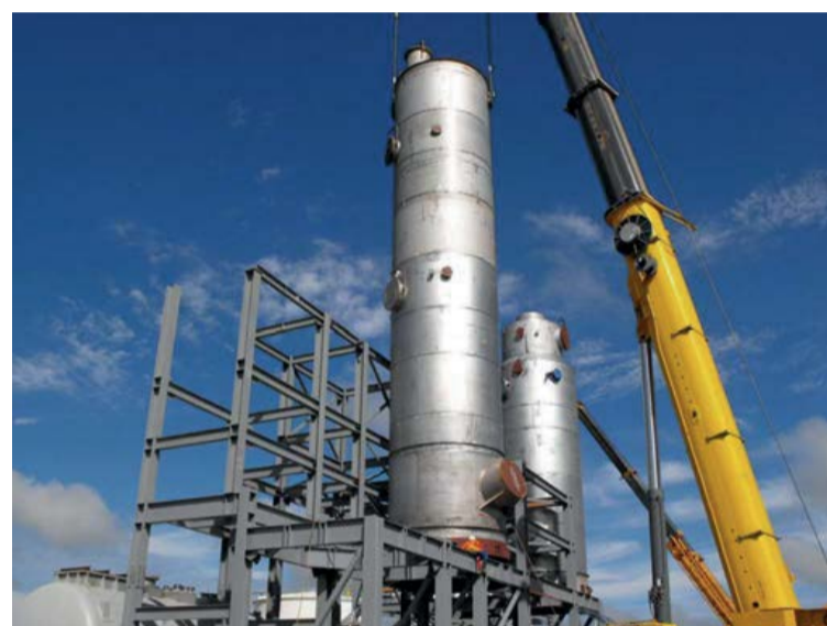
Fig. 5: SARAMET® acid towers lifted into position.
