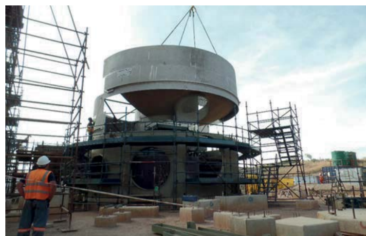
Fig. 3: Converter modules assembly in-field.
