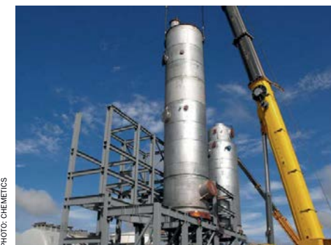
Fig. 5: SARAMET® acid towers lifted into position.
