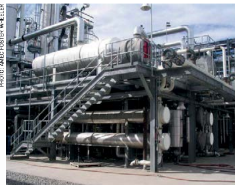
Fig. 2: View of modular installation, note lower module structure is covered by finished concrete.
