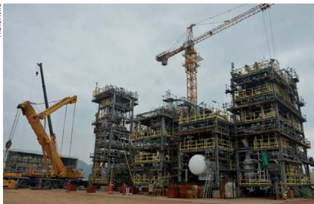
Fig. 1: RATE modular design for a sulphur recovery unit.
