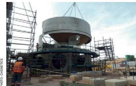
Fig. 3: Converter modules assembly in-field.
