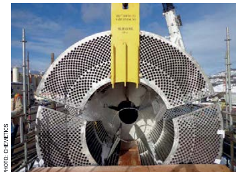
Fig. 10: Assembly of segmental tube bundle exchanger on site.
