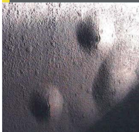
Fig 10: Hydrogen-induced cracking and blistering
