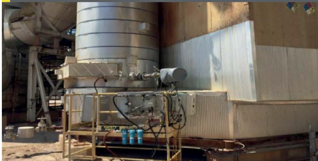
Fig 6: AbSensor-ADM-SA installation
