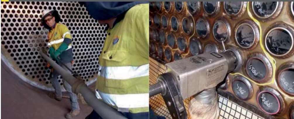
Fig 5: Insertion (left) and cutting (right) of new tubes
