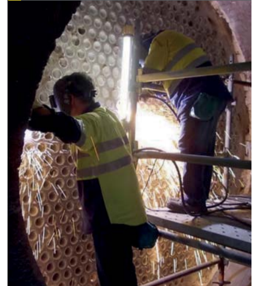
Fig 4: Hot end tube cutting
