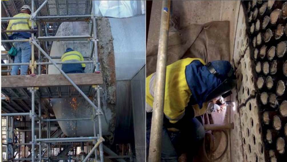
Fig 3: Cutting WHB cold end vestibule (left) and tube sheet (right)
