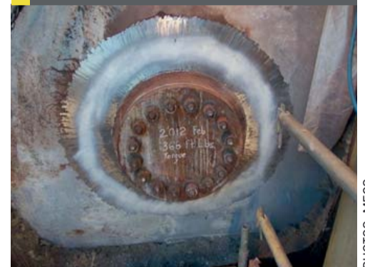
Fig 6: Marking out hand holes prior to complete removal
