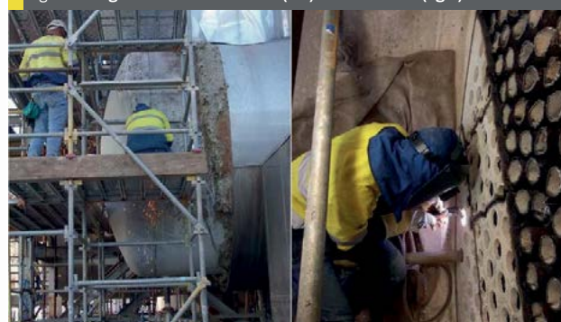
Fig 5: Insertion (left) and cutting (right) of new tubes
