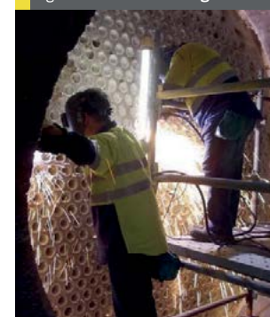
Fig 6: Marking out hand holes prior to complete removal
