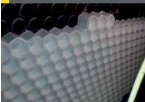
Fig 10: IPL Mount Isa ferrule installation with HexPro™ ferrules
