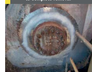
Fig 6: Marking out hand holes prior to complete removal
