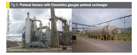
the converting step), the catalyst temperature will drop which will result in high  $SO_2$  emissions. Chemetics preheat furnace system is designed to heat up from ambient to >700°C in less than 15 minutes. This is achieved through specialised furnace refractory design and use of Chemetics patented radial tube stainless gas-gas heat exchangers (Fig. 6)
