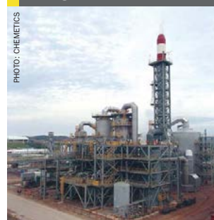
Fig 10: Sulphuric acid plant with tail gas caustic scrubber
