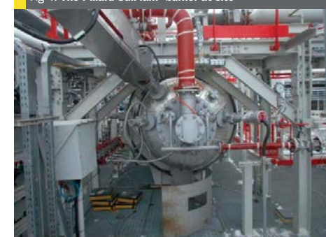
Fig 4: The Pillard SulFlam® burner at site
