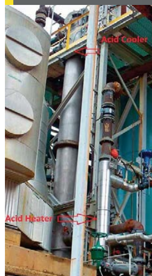
Fig 13: Insulated NORAM acid warm-up heater installed in parallel to the horizontal acid cooler
