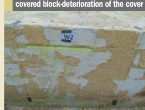
Fig 9: Vertical side stucco concrete covered block-deterioration of the cover
