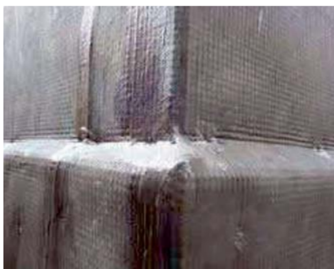
Fig. 7: Prefabricated seamed and sealed fabric reinforced waterproofing membrane.
