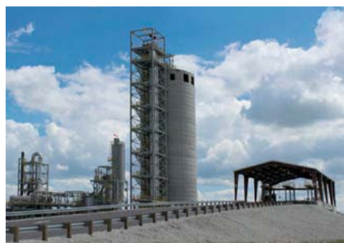
The finished New Wales melter
