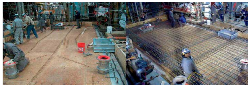
Fig. 5: Sleeved process piping penetrations and entry portals positioned prior to sulphur pit roof slab concrete placement.
