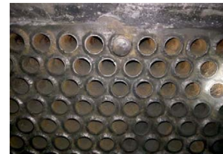
Fig. 2: Aluminised tube sheet after cleaning.
