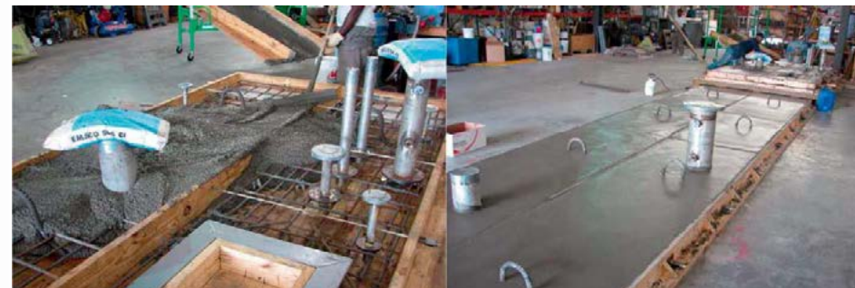
Fig. 6: Precast concrete sulphur pit roof slab panels that incorporate “spool” penetrations installed during concrete casting/placement.
