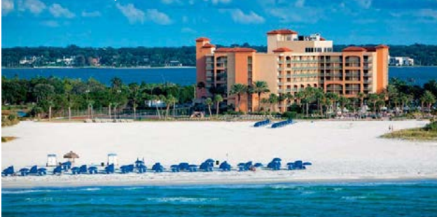
The Sheraton Sand Key resort, Clearwater, Florida.
