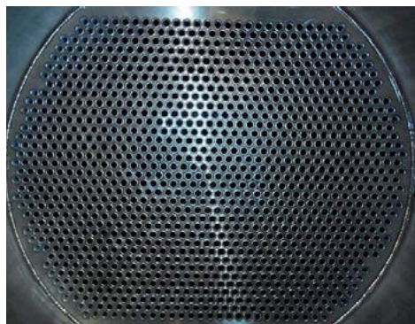
Fig. 5: MECS ® ZeCo ® acid cooler tubesheet.
