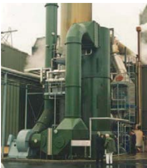
TurboScrubber installation.
