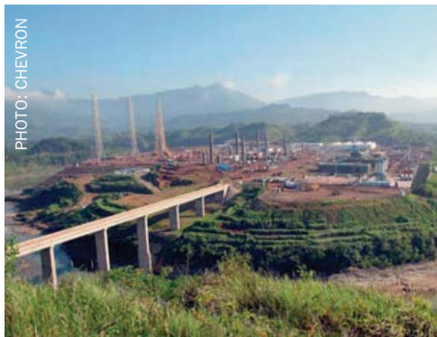
PHOTO: CHEVRON Luojiazhai gas plant.
