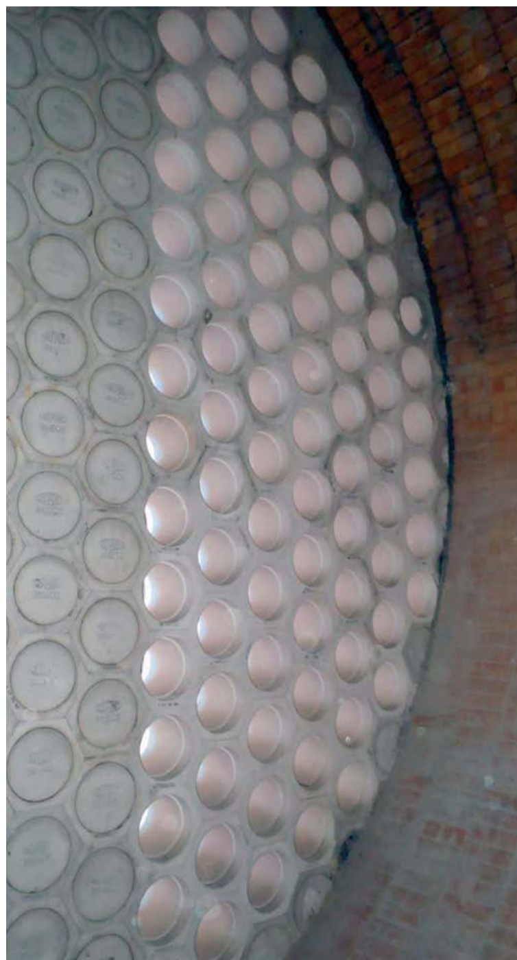
Furnace replacement at DuPont, Burnside, Sulphur 356, Jan/Feb 2015, p52.
