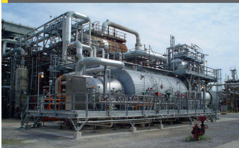
Fig 5: SRU thermal train
