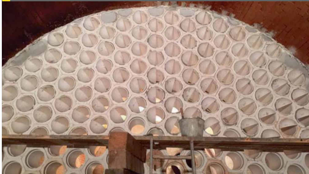
Fig 8: Recent VectorWall™ installation for narrower residence time distribution
