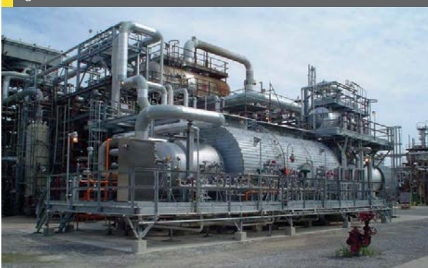
Fig 5: SRU thermal train
