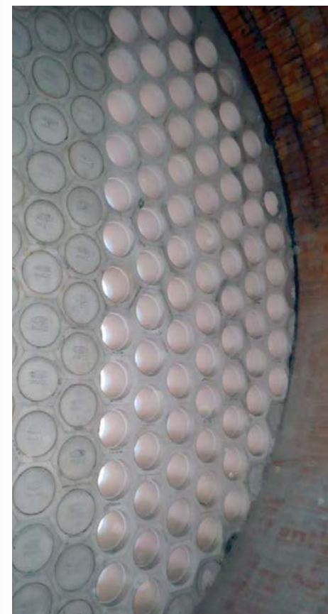
Furnace replacement at DuPont, Burnside, Sulphur 356, Jan/Feb 2015, p52.
