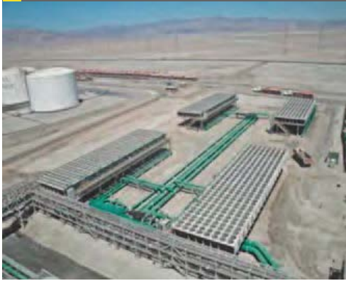
Fig 11: Fin-fan closed loop water coolers
