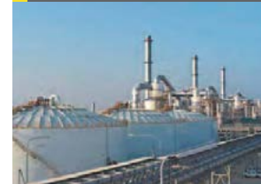
Fig 4: The world's largest single train sulphuric acid plants
