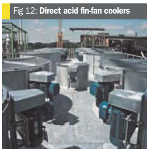
Fig 12: Direct acid fin-fan coolers
