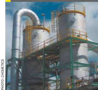
Fig 3: Design models for these acid towers were confirmed using plant data
