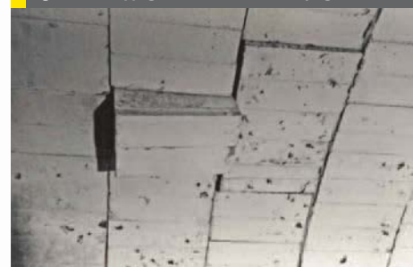
Fig 5: Brick slippage due to insufficient keying action
