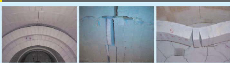
Fig 4: Classic examples of high temperature deformation
