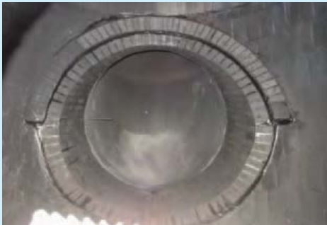
Replacement of the gas inlet nozzle of an existing absorption tower: after removal of the brickwork in the intermediate zone, the damaged nozzle was cut off and replaced.
