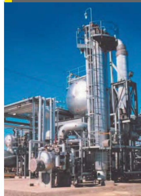
Fig 9: The D'GAASS unit has a pressurised vertical vessel
