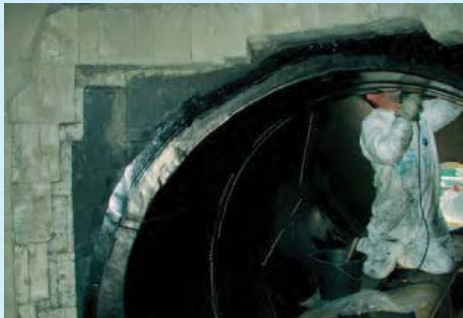
Replacement of the gas inlet nozzle of an existing absorption tower: after removal of the brickwork in the intermediate zone, the damaged nozzle was cut off and replaced.
