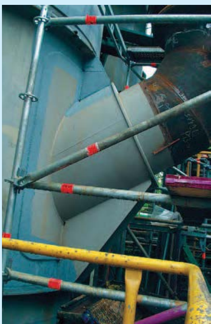
Replaced gas inlet.
