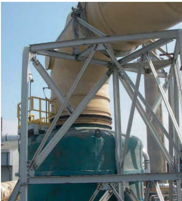
FRP is widely used for duct work.
