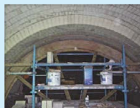
To reduce the production loss, the bricklining job for a new furnace took place beside the plant while the existing combustion chamber was still in operation.
