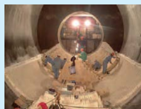
To reduce the production loss, the bricklining job for a new furnace took place beside the plant while the existing combustion chamber was still in operation.
