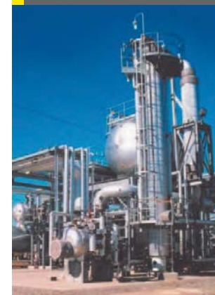
Fig 9: The D'GAASS unit has a pressurised vertical vessel
