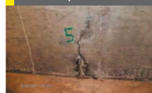
Fig 11: Sulphur pit cracks before start-up
