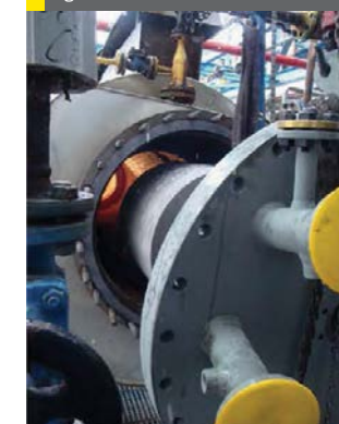
Fig 3: Fit out of a tested burner
