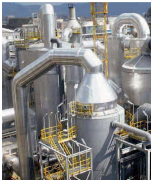
Tsumeb acid plant.
